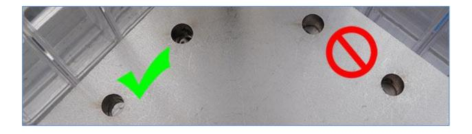
To avoid this problem, leave the floor profile connector fasteners loose and adjust for perfect hole alignment. Inconsequential gaps might appear between the edges of the floor profiles and the plastic corner connector.
