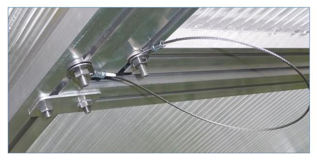
Two restraints are used for each window; one on each side. Install each loop between two flat washers on screws that were loaded in Steps 1 and 11. Position the restraint as illustrated and adjust as needed to avoid interference from the crossbar as the window is raised and lowered.
