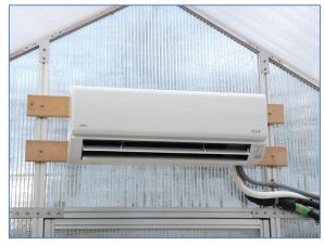
Ductless mini-split heat pump indoor unit
