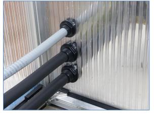
Glazing penetrations for refrigerant lines and power
