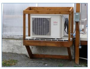
Ductless mini-split heat pump outdoor unit
